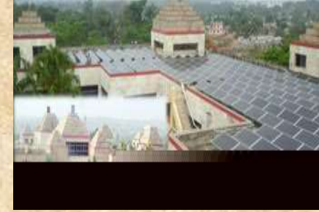
SOLAR POWER PLANT
