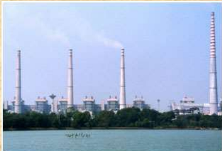
CAPTIVE POWER PLANT
