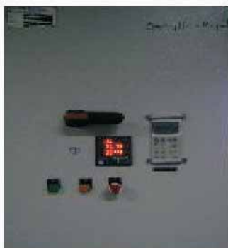
Installation of VFD at cooling water pump 2 motor in pm2
