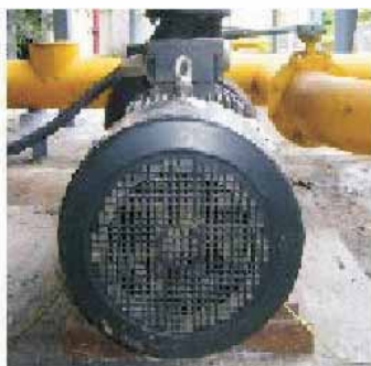
Replacement of old inefficient condenser pump2 with energy efficient pump2
