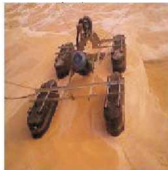
Installation of Titon Aerator in ETP -1 No
