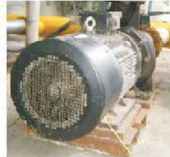
Replacement of old inefficient condenser pump1 with energy efficient pump
