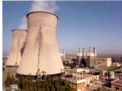
In combined cycle operation, the exhaust is diverted through a diverter damper assembly into a waste heat recovery boiler. Each of the gas turbine is provided with a waste heat recovery boiler which discharges flue gas through 55 M high boiler stacks.
