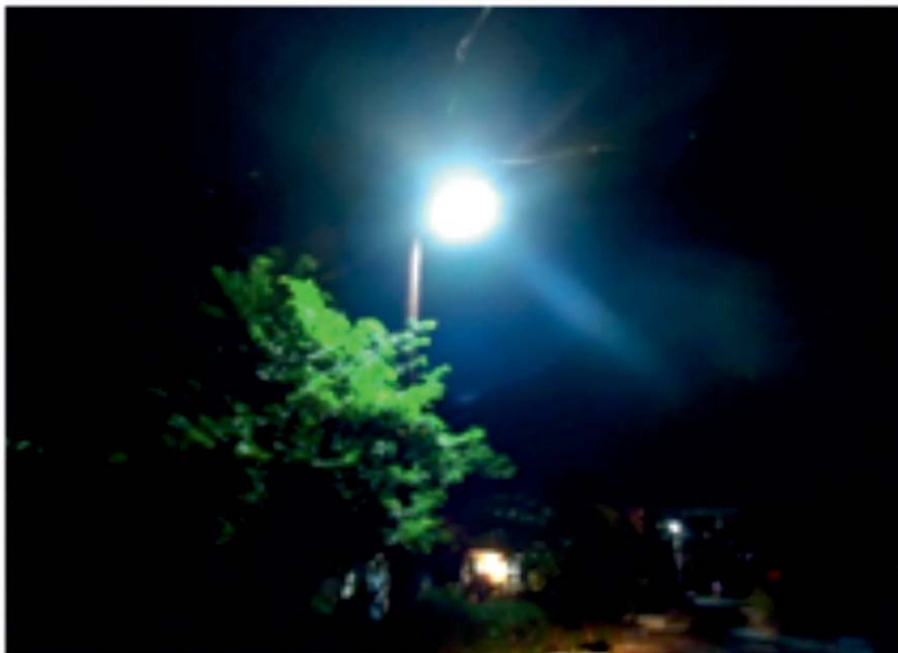
Installation of LED Street Lighting
