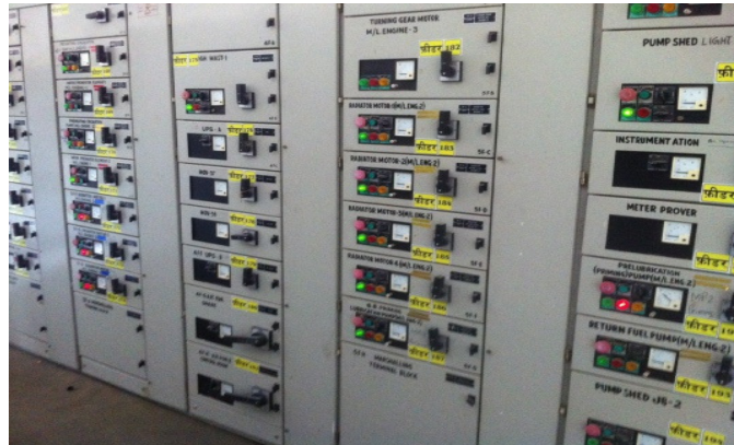
ELECTRICAL SWITCH YARD
