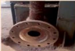
Eliminated header gasket failure of FBC boiler by replacing the steam header's hand hole plate with Flanged plate. Improved FBC boiler availability and reduced HSD boiler running hrs.
