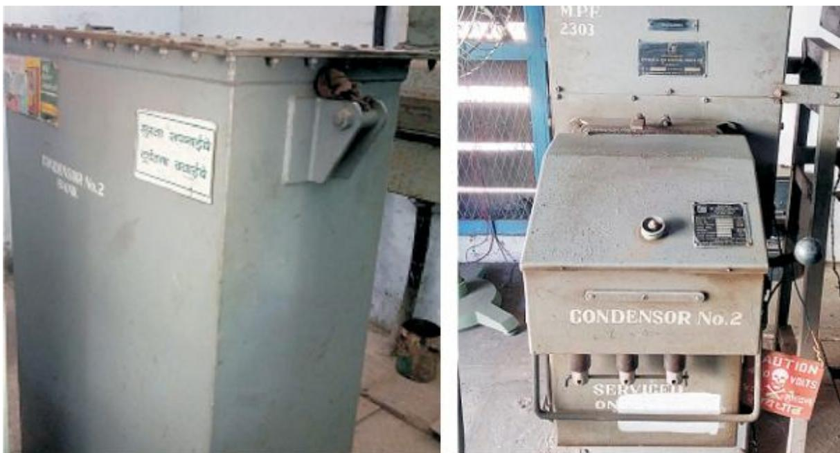
155 KVAR Static Condensor Bank with switch in OFF Condition
