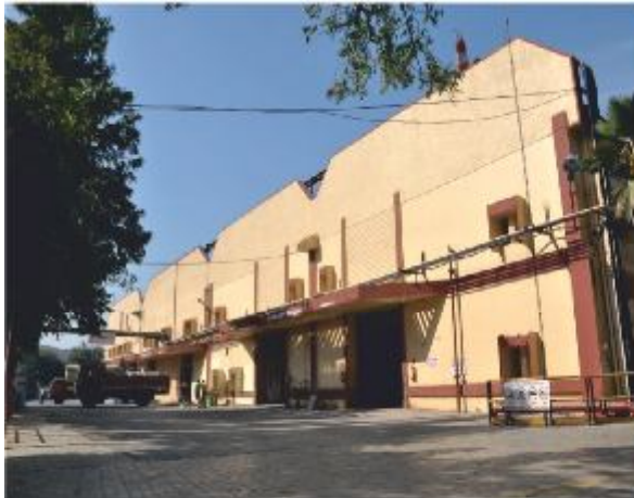
Solvent & Water Base Plant
