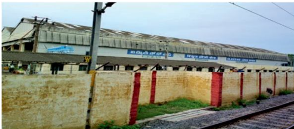
Electric Loco Shed, Kazipet
