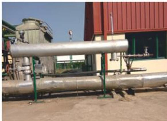
Project-5 Flash Steam recovery from Process house steam condensate tank:
