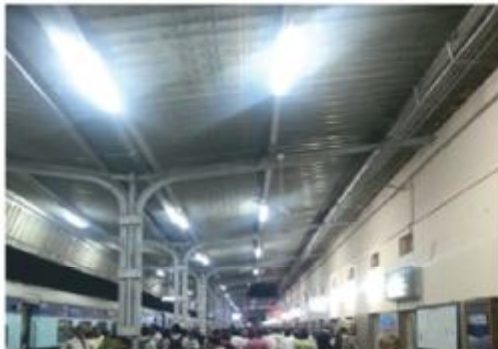
100% LED at Nizamabad Station
